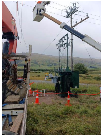
Field verification, December 2025. Site rated Excellent; isolation, MADs, working at heights and lifting separately verified, with photographs at each.
